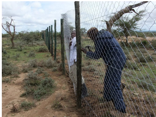
Building The Fence
